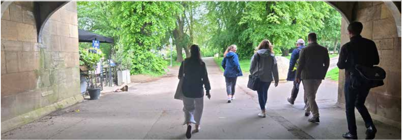
Figure 79 Wide footpaths under Skeldergate Bridge
