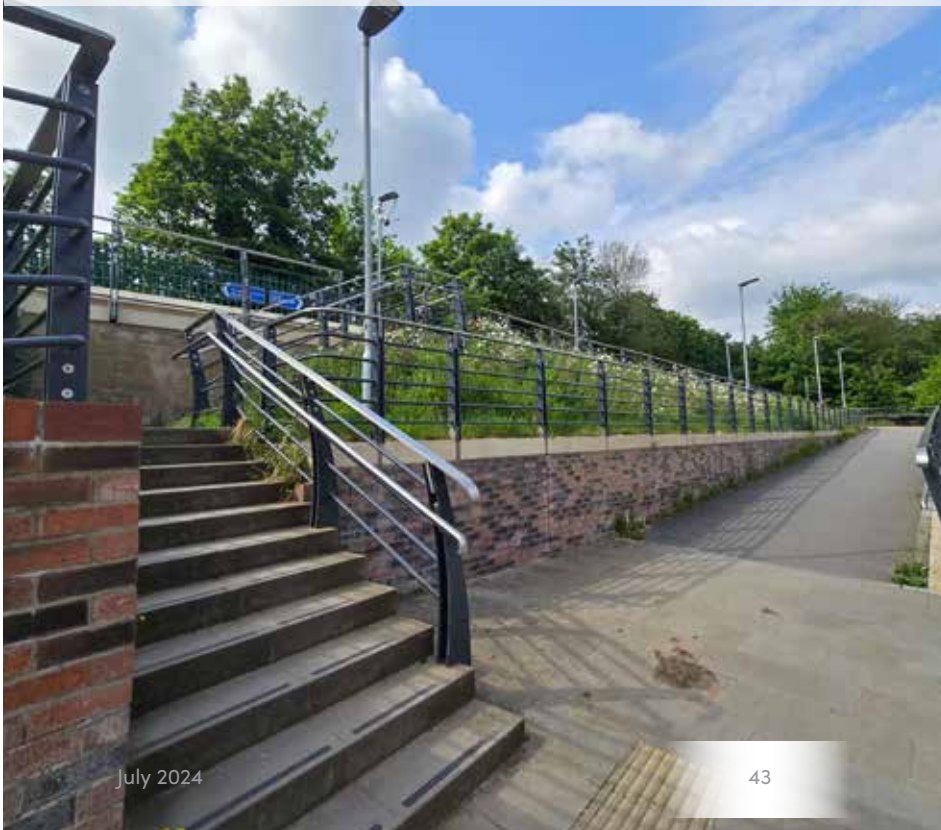
Figure 89 Stepped and ramped access to Scarborough Rail Bridge
