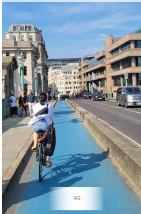
Figure 182 Full segregation on the Cycleway 7, Southwark Bridge (Southwark)
