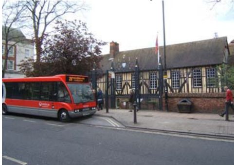
Stops can detract from historic buildings
