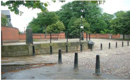
Badly designed areas beside the river and Yorkshire Museum Gardens
