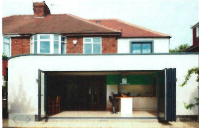
Contemporary extension on Hunters Way (ground and first floor render)
