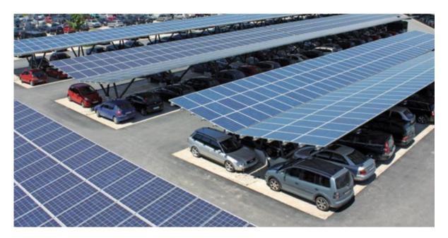
17. Above is an image of what the solar canopies would look like. The canopies would use the free space immediately above the vehicles to harvest solar energy to the site. Batteries would then store the electricity,
